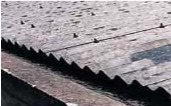
Figure 1: Asbestos Cement Roofing Sheets
